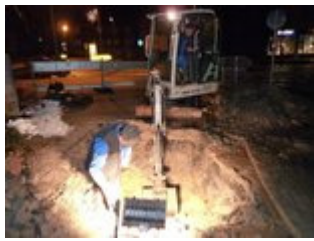
Wasserrohrbruch in Altenberge
